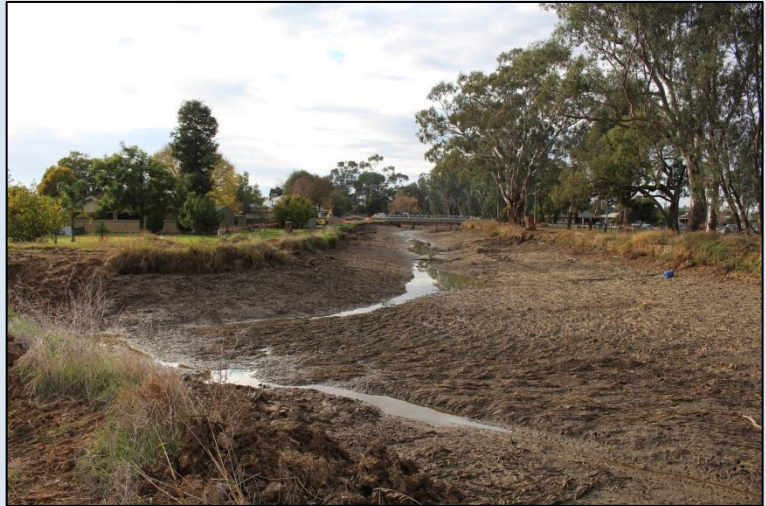
A photo taken of the irrigation channel before operations had begun on this area.
